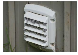
Now that we've covered the importance of why you need to clear the vent, let's go over how exactly to do it. Here's a simple step-by-step guide on how to unclog your dryer vents:
